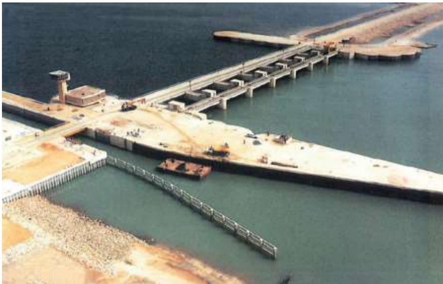
Figure 102. Barrage de Diama (source : Artelia)
