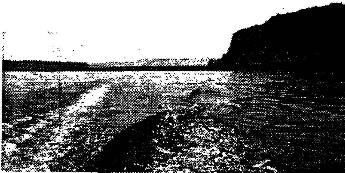
Figure 9. Right abutment of Manantali Dam from upstream, along northeastern shore of reservoir. Also see Figure 10. Photo by Leeds.
