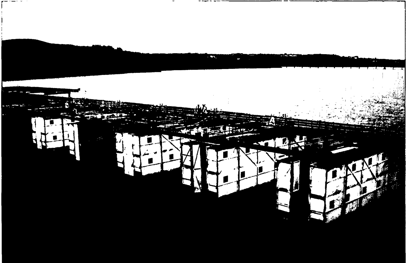
Fig. 4: Enclosures around pile bents
