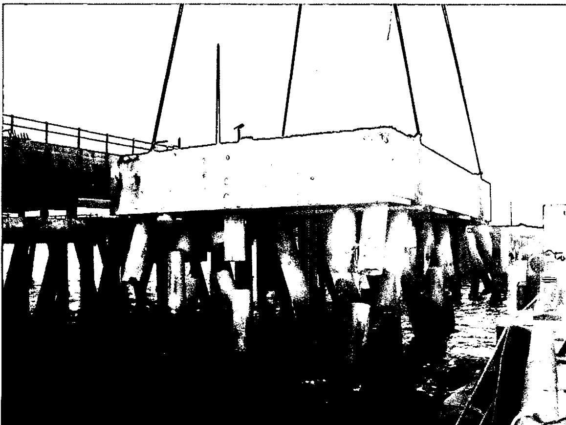
Fig. 6: Lifting of mooring dolphin pilecap after cutting piles
