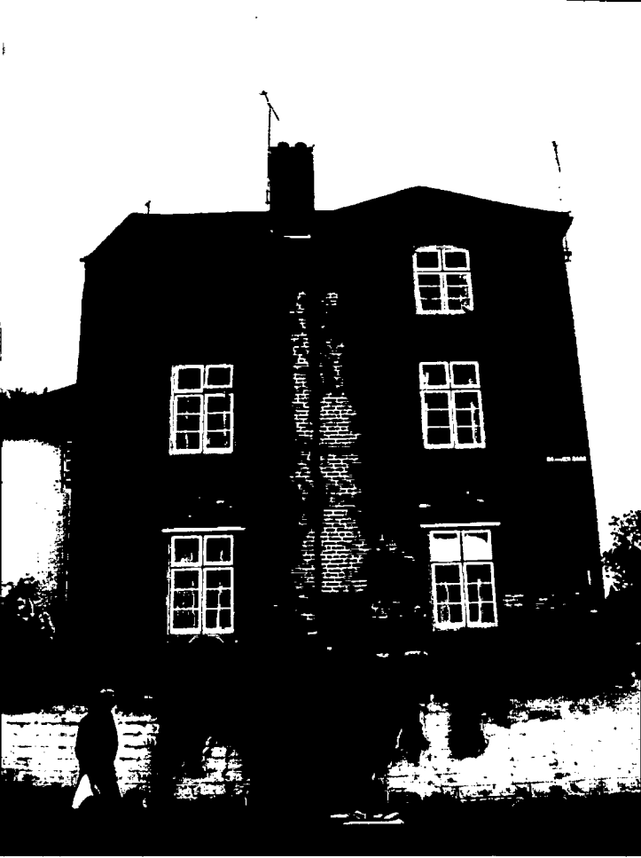
Fig. 6: House in Severnside before restoration in 2004
