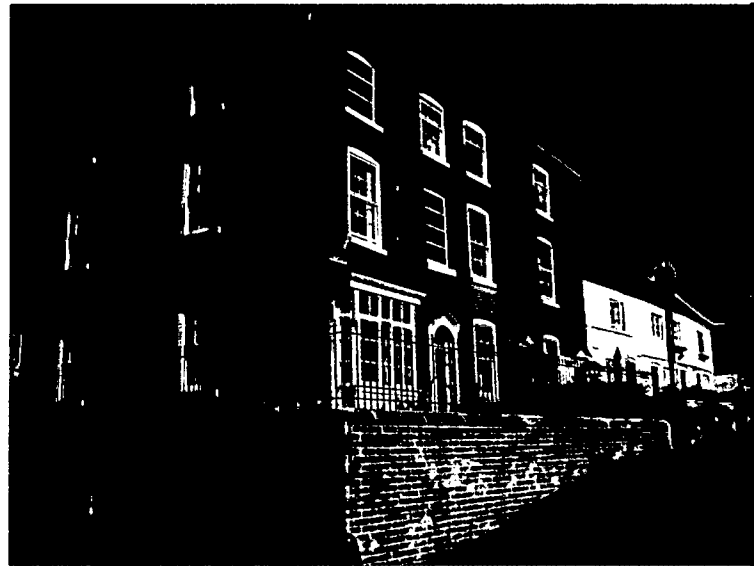
Fig. 7: House in Severnside after restoration in 2007
