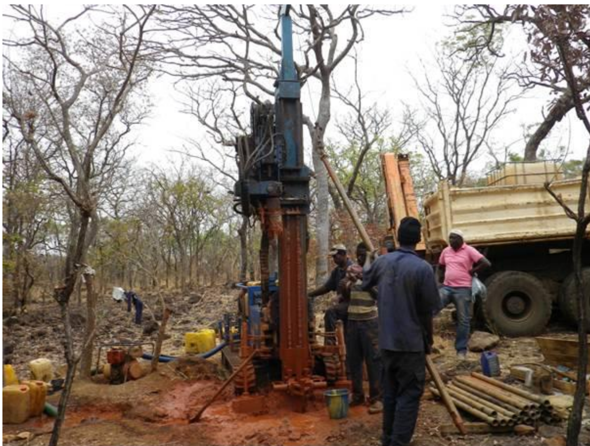
Figure A2. 31 – Campagne de reconnaissances de TRACTEBEL Engineering (2011-2012) – Perforation du sondage S1
